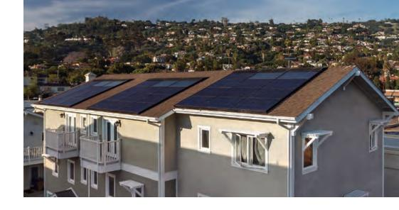
taped, sealed, and caulked gaps around every piece of drywall, window, door, wall penetration, and siding, air leakage was kept to a minimum. Together, they helped the project achieve Passive House certification, the first multi-family development in Southern California to do so.
