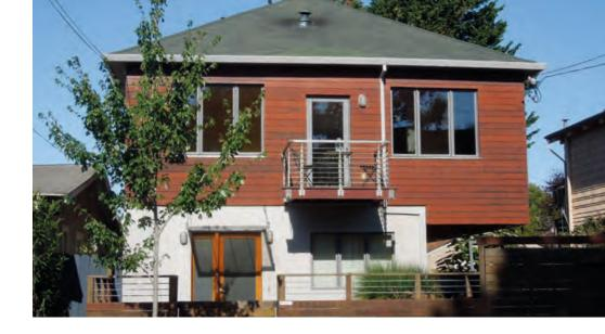
Due to the mild Berkeley climate, the PHPP indicated that 2 x 6 stud walls with cellulose insulation and 2 inches of exterior rigid insulation would be enough to meet the Passive House standard. The heat-recovery ventilator made a significant difference. The biggest challenge, especially then, was to convince the construction team of the importance of air sealing. After implementing several techniques, the final blower door test measured 1.1  $ACH_{50}$ .
